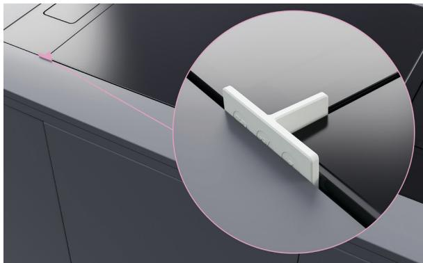
**1. Slot the T spacers between the products. Adjust positioning to ensure even spacing between products is achieved.**
