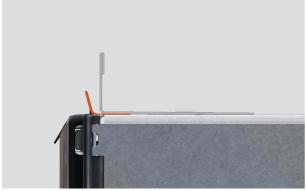
**3.** Ensure the front of the rubber seal is free of the bracket.
