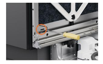
1. Fit a screw in each chassis slot to secure to the cabinet. Partially tighten screws ensuring adjustments can be made.
