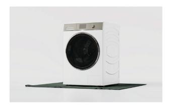
Protect flooring before positioning products as close to the installation location as possible, ensuring enough working room is left available.
