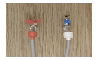
15. Connect hoses to taps before turning on. Check for leaks at all connection points. If possible, recheck for leaks 24 hours after installation.
