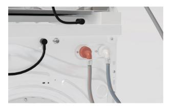
10. Connect the angled end of hot hose to the orange outlet on the washer. If hot hose is not required, install a blanking cap.
