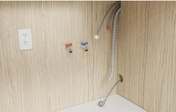
5. Route the power cables and hoses through service holes.
