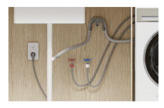
**9.** Connect the power cable and check washer is powered on and connected.
