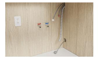
**5.** Route the power cables and hoses through service holes.
