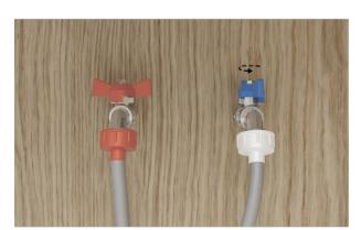
9. Connect the cold hose to cold water tap and turn tap on. If possible, recheck for leaks 24 hours after installation.
