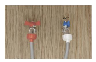
**8.** Connect hoses to taps before turning on. Check for leaks at all connection points.
