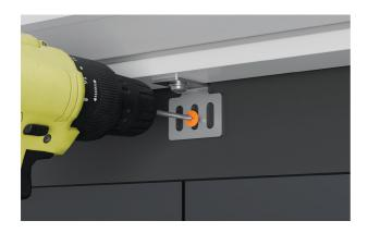
**2.** Fit an additional screw through the bracket to lock panel into position.
